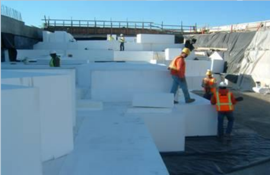
I-680 Interchange – Martinez, CA
