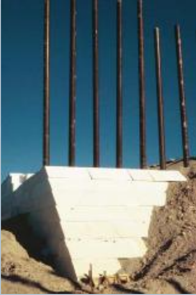
Bridge Abutment With Piles
